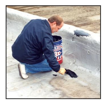
WINTER-PATCH PLASTIC CEMENT is a trowelable, asphalt-based, cold weather roof repair compound. It may be used with GLAS-WEB Roofing Mesh to add even greater strength and life to your roof repairs when weather, temperature and exposure time allows.
