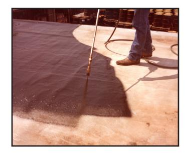
MIGHTYPLATE Roof Coating is a cold process asphalt-base coating. It preserves and prolongs the life of a roof by creating a seamless, pliable, long-lasting layer of water-repellent protection over existing roof surfaces. Engineered to rigid quality control specifications. After 70 years of use - MIGHTYPLATE Roof Coating has proven to be a very successful, consistent performer. MIGHTYPLATE Roof Coating can add years of service to a roof investment.
